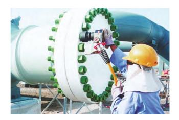
including the design of tightening procedures, advice on preferred equipment to be utilized, on the job installation and tightening, and post job reporting. Our highly skilled technicians use their in-depth technical knowledge and best industry practices to ensure accurate bolt loading is achieved. We pride ourselves on the belief that our hydraulic torque equipment is the safest and most advanced equipment used within the service industry.
